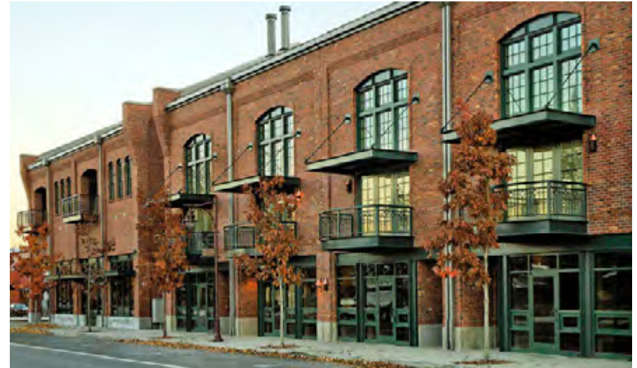
Figure A.20 Here, projecting balconies are used to modulate the facade of building longer than 50 feet.
