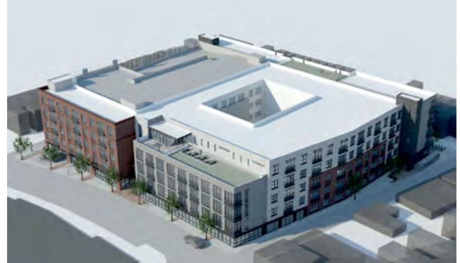
Figure E.4 An example of a parking garage shielded by housing and mixed use building liners.
