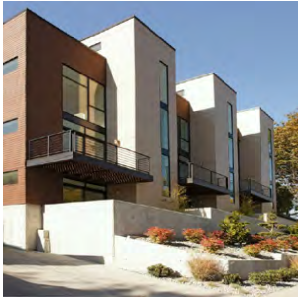
Figure A.9 An example of a vertical material change that occurs on an alternate or offset plane.
